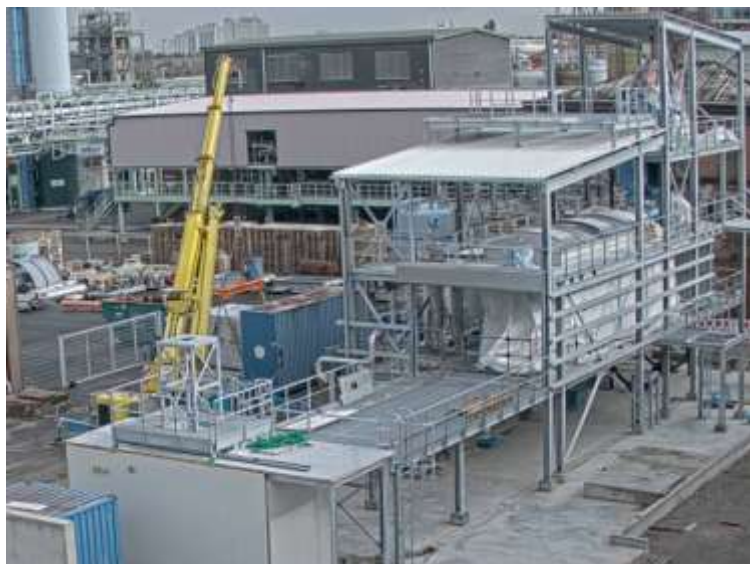
Location at Industrial Park Höchst (in construction)
